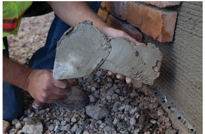
The mason must completely back butter the entire unit.
