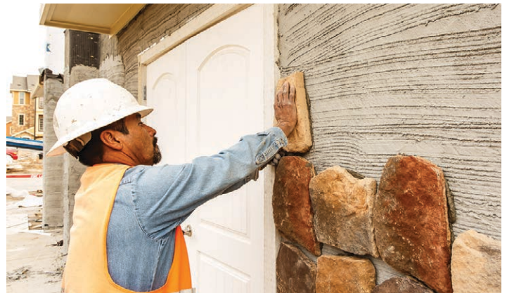
Shown is a thin natural stone veneer unit being installed.
