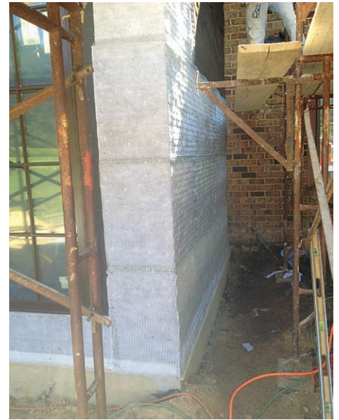
Shown is installed Lath Net, ready for the scratch coat.
